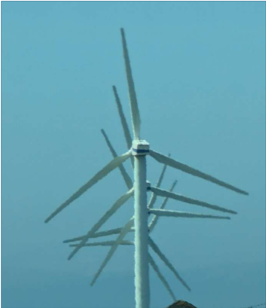
Wind turbines on Cumbria Coast, Image credit: Irish Sea Rim
